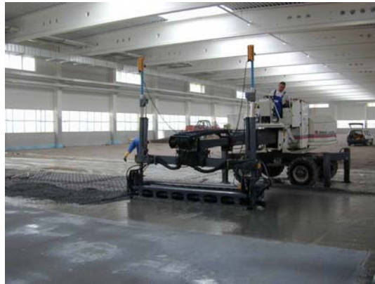
Fig. 4 Secondary barrier / Laser screed compacting and levelling concrete
