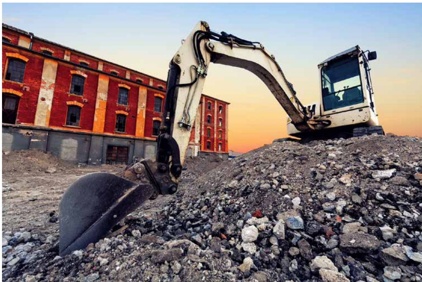
fig: practical application demonstration of recycled constituents in precast construction
